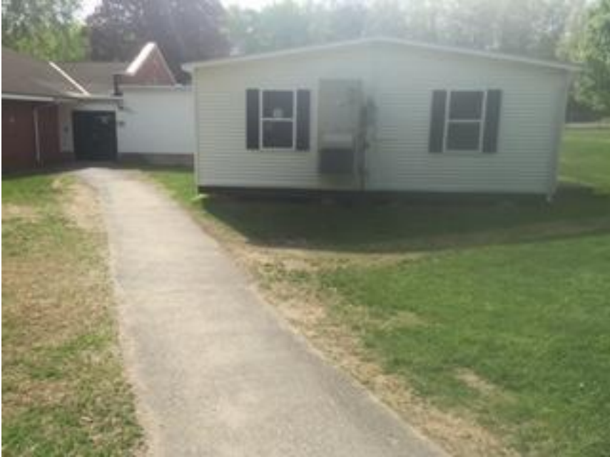
Hallway connecting existing unit to main building
